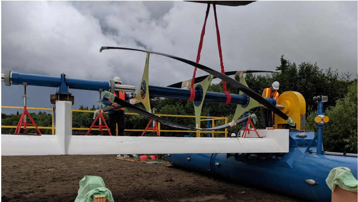
Figure 11. Installation of the first RivGen turbine onto the mid-stanchion
