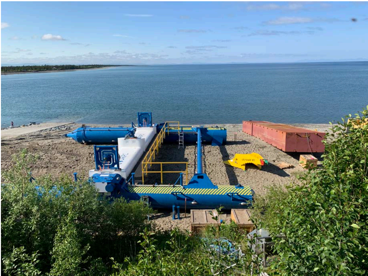
Figure 7. Re-assembly of the RivGen device major structural components
