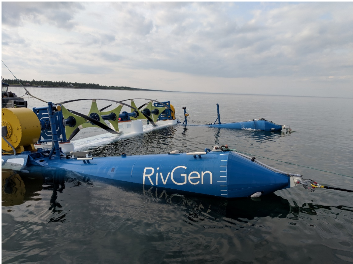
Figure 23. Retrieval attempt using secondary buoyancy system and "all chambers" evacuation, which resulted in "bow up" orientation that prevented full retrieval, highlighting the risk of an “all chambers” evacuation
