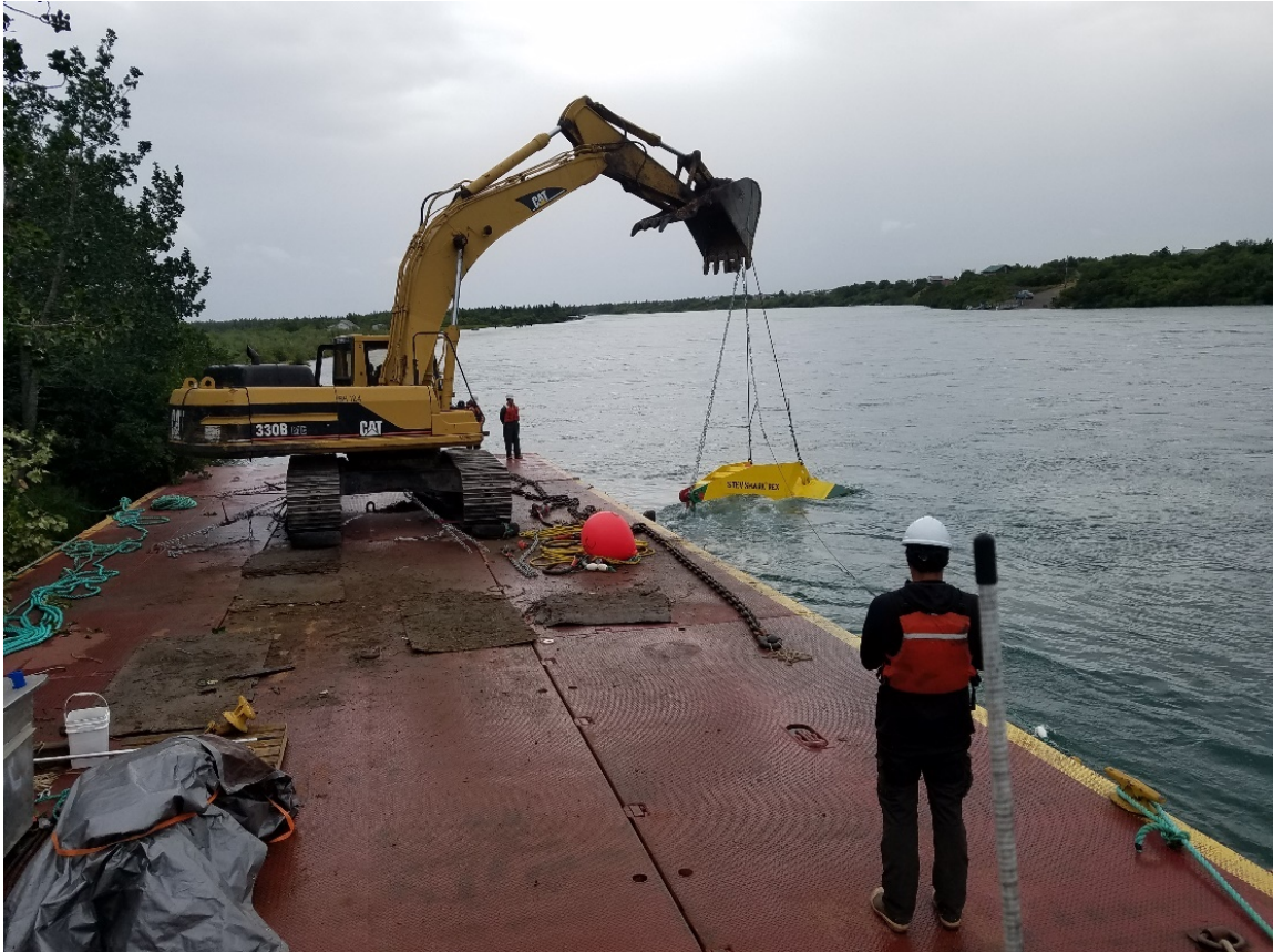
Figure 18: Anchor installation tests using modified install approach
