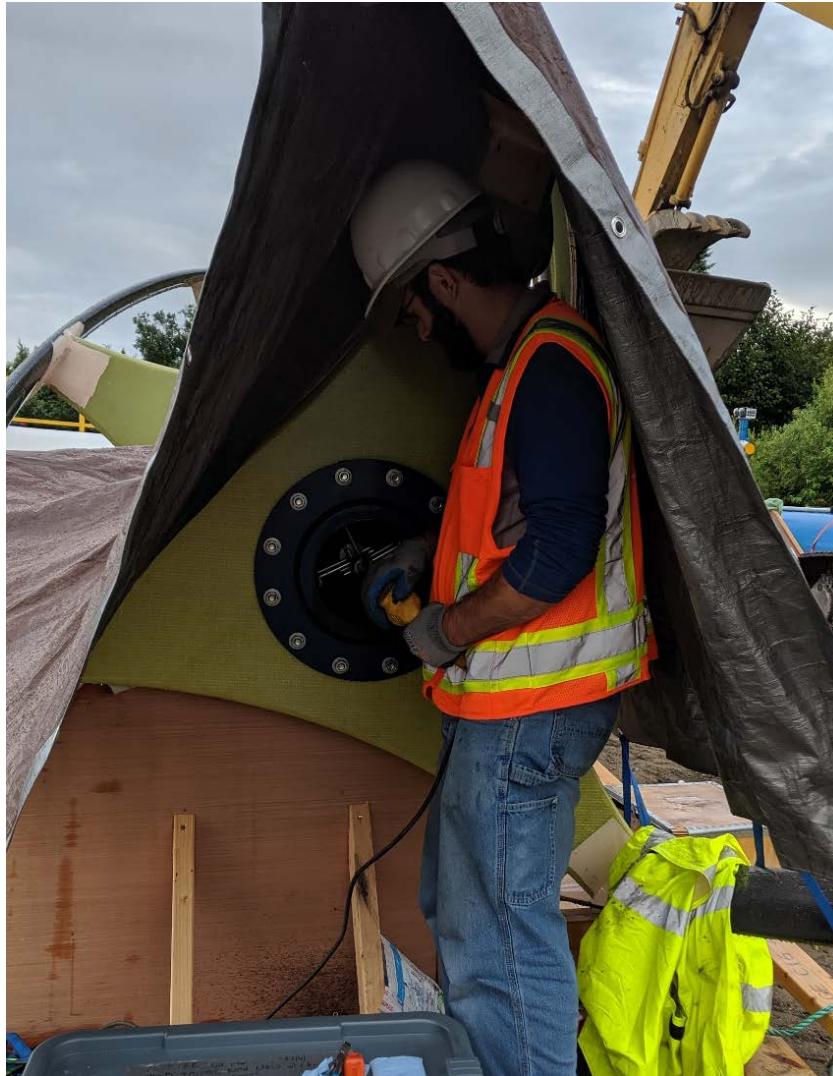
Figure 10. To correct tolerance issues on the turbine shaft ID a cylinder hone was used.
