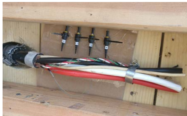
Figure 34. Exposed Fibers (the four fiber terminations above the main cables with the exposed fibers extended below the main cable) at the submarine P&D cable shore-side termination
