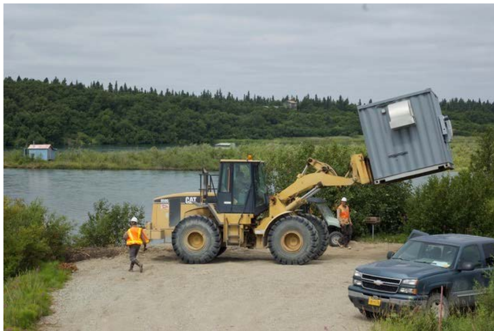
Figure 13. The shore station was moved to its installed location.
