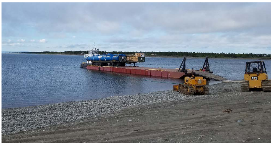
Figure 6. Offloading the RivGen Power System at Igiugig
