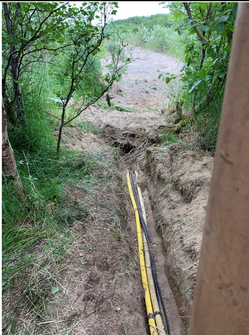
Figure 16. Terrestrial P&D cable installation
