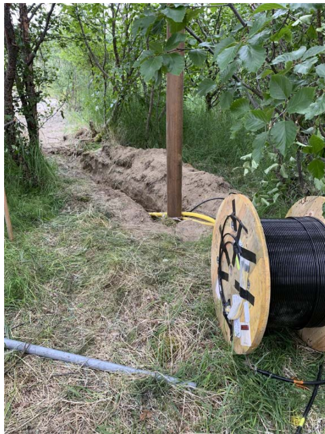
Figure 14. Junction box mounting pole installation
