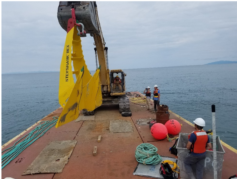
Figure 17. Preliminary anchor lifting/deployment test
