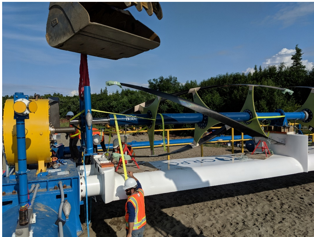
Figure 12. Installation of the end stanchion onto the second turbine
