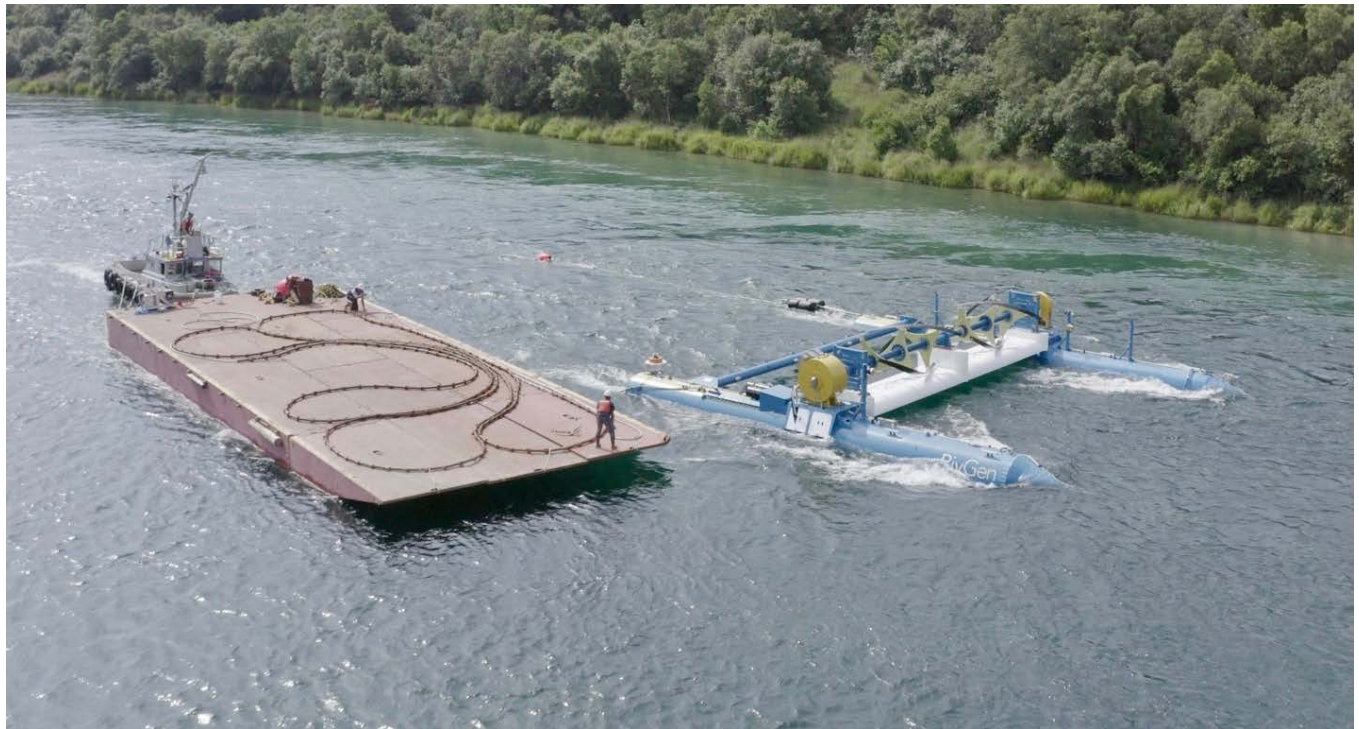
Figure 32. P&D cable installation
